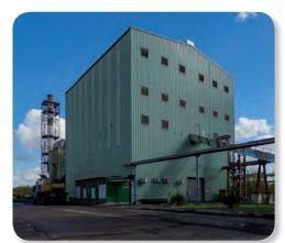
Since 2008, all bark and wood waste, together with sludge from treatment facilities, are incinerated to obtain heat energy in a powerful Wellons boiler (USA), and the ash formed as a result of waste incineration is cooled and utilized without posing a threat of pollution to the environment.
